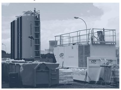
CTP environnement deployed a **Clearflow**® mobile unit to minimise the foaming (emulsifying) properties of the effluent. This physico-chemical treatment, combined with an activated carbon filter, was designed to eliminate as many pollutants as possible before discharge to the plant's biological treatment plant. This plant was not able to process such a large load impacting its performance and therefore compliance with discharge standards being put at risk
